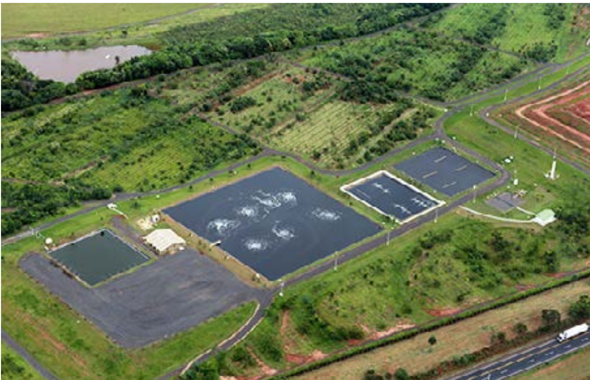
Water treatment plant (WTP). Bacía do Rio Grande (Brazil)
