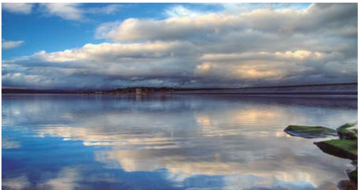
Valmayor Dam (Community of Madrid, Spain)
